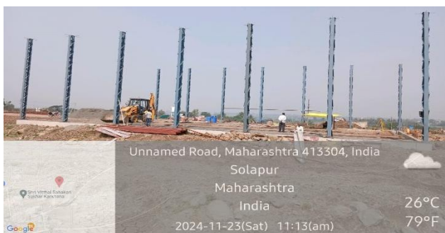
Mechanical Work at CBG Plant
